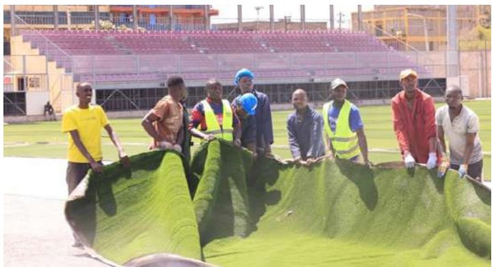
Ongoing construction works at the Dandora Stadium
